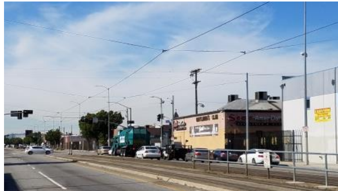
Figure 13: Blue line trolley wire & cross wire
